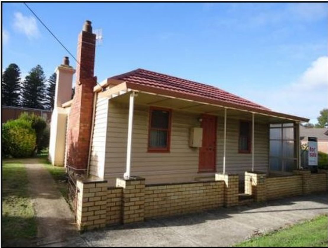
The original weatherboard cottage at 40 Lava St, previously owned by Lottie Bowman. Image: Justin Allen, Northeast, Stockdale and Leggo real estate.
