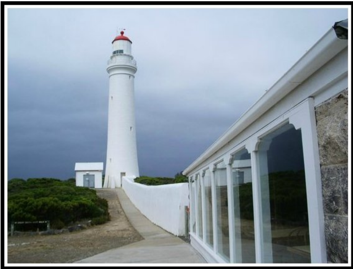
The imposing lighthouse and refurbished frontage of Isabella's cafe which
